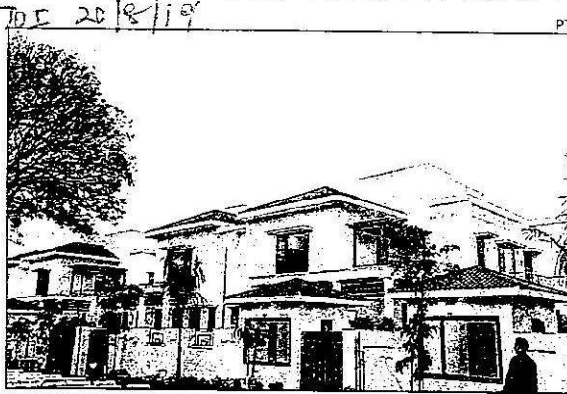
HOUSING LAWMAKERS: PM Narendra Modi inaugurated 36 duplex flats for MPs at North Avenue in New Delhi on Monday
