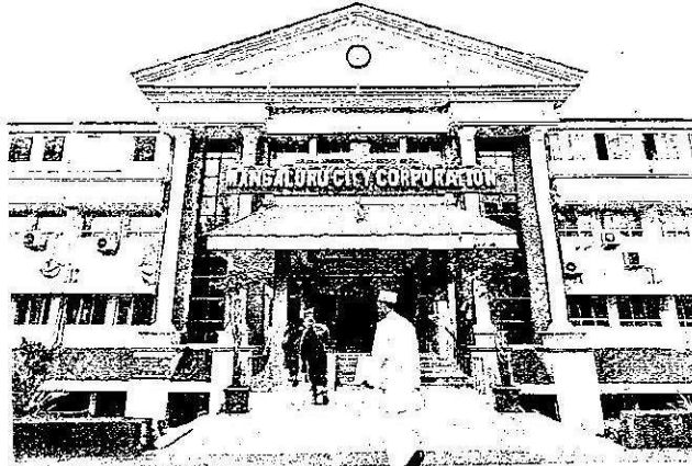
A view of Mangaluru City Corporation building.
