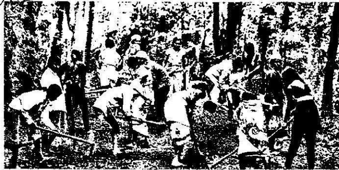
Villagers carry out road-laying work near Terali village in Uttara Kannada | DHEMANTH
