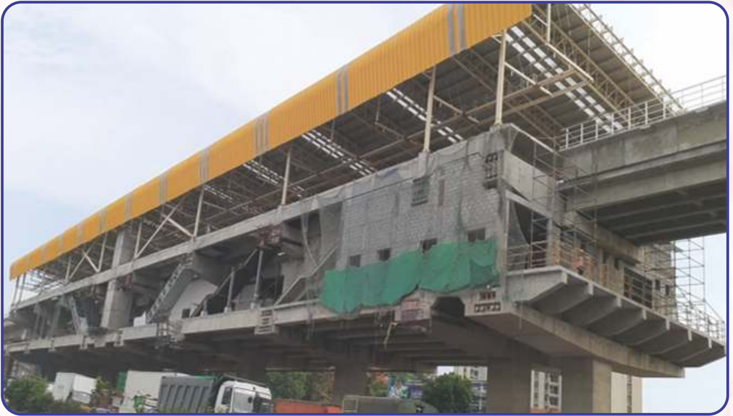
Reach 5 (Package 1) Huskur Station works in progress
