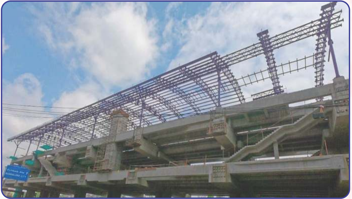
Reach 1A: Benniganahalli Station Roof portal erection work in progress
