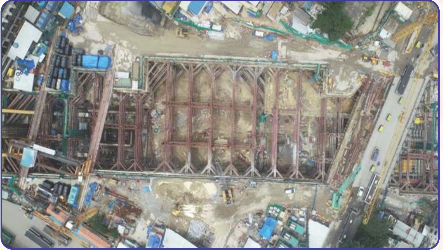
Reach-6 (UG) Aerial View of Shivajinagar Station
