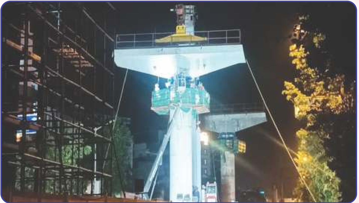
Phase 2A/Package-2 - Pier Cap Erection
