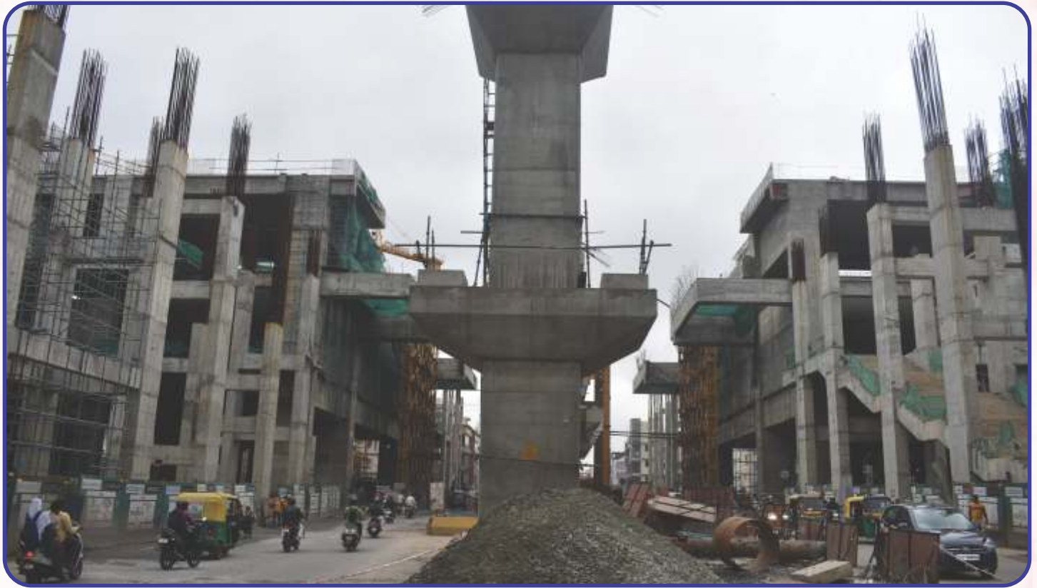
Ongoing works at Jayadeva Metro Station
