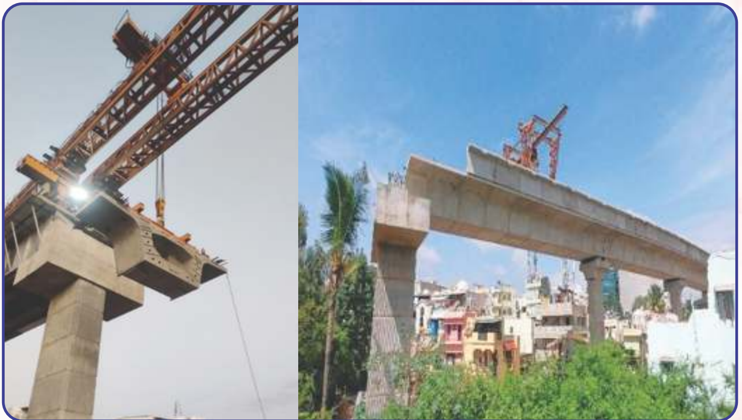
Reach 1A: Segment & Parapet erection work in progress
