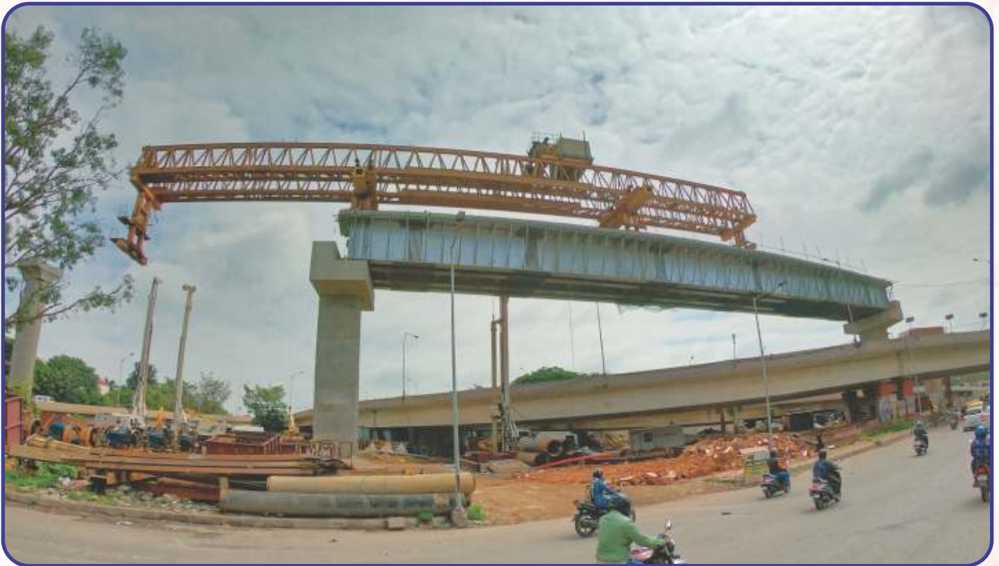
Metro Pier ID BP31-BP33 (Near Benninganahalli Lake)
