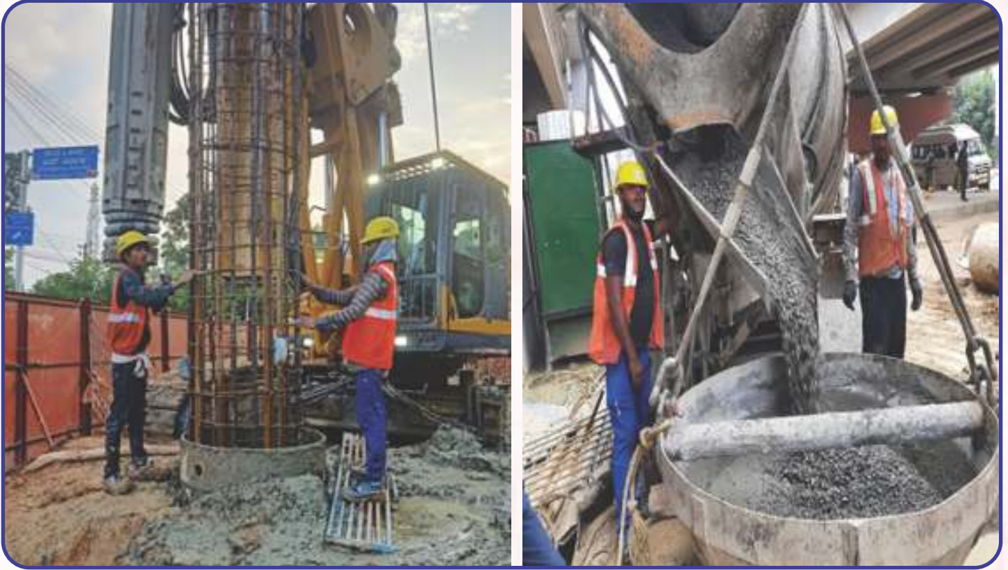
Phase 2A/Package 1 - Viaduct Pile Concreting work is in progress
