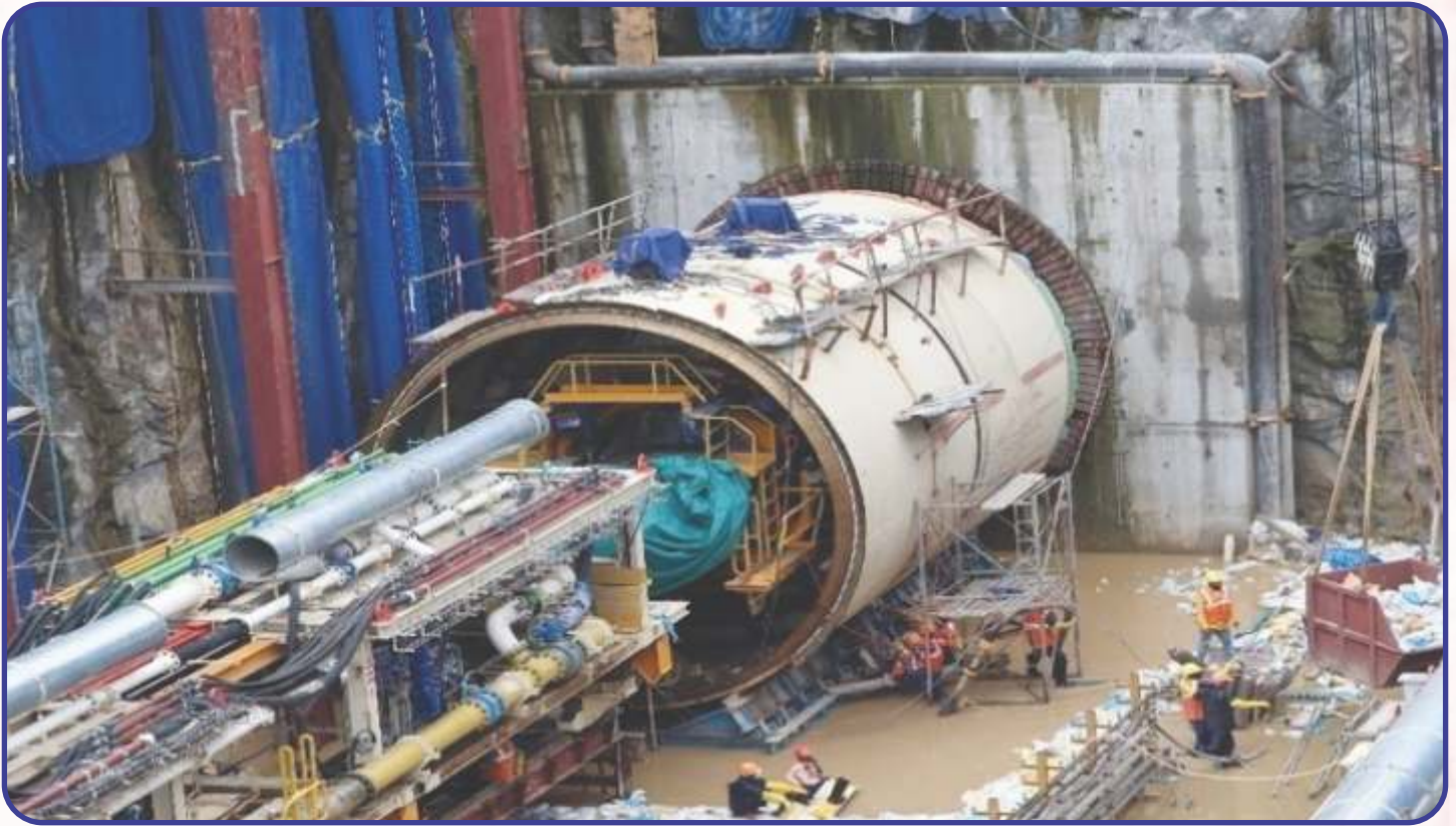
Reach-6 (UG) TBM Vindhya Commissioning
