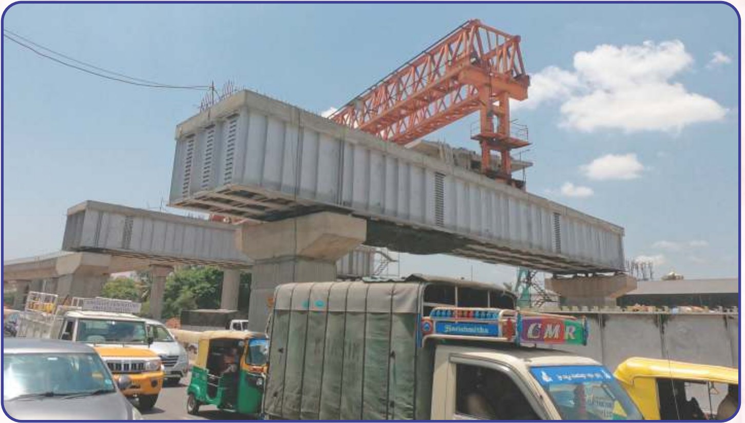
Metro Pier ID BP47-BP48 (Near Tin Factory Junction)
