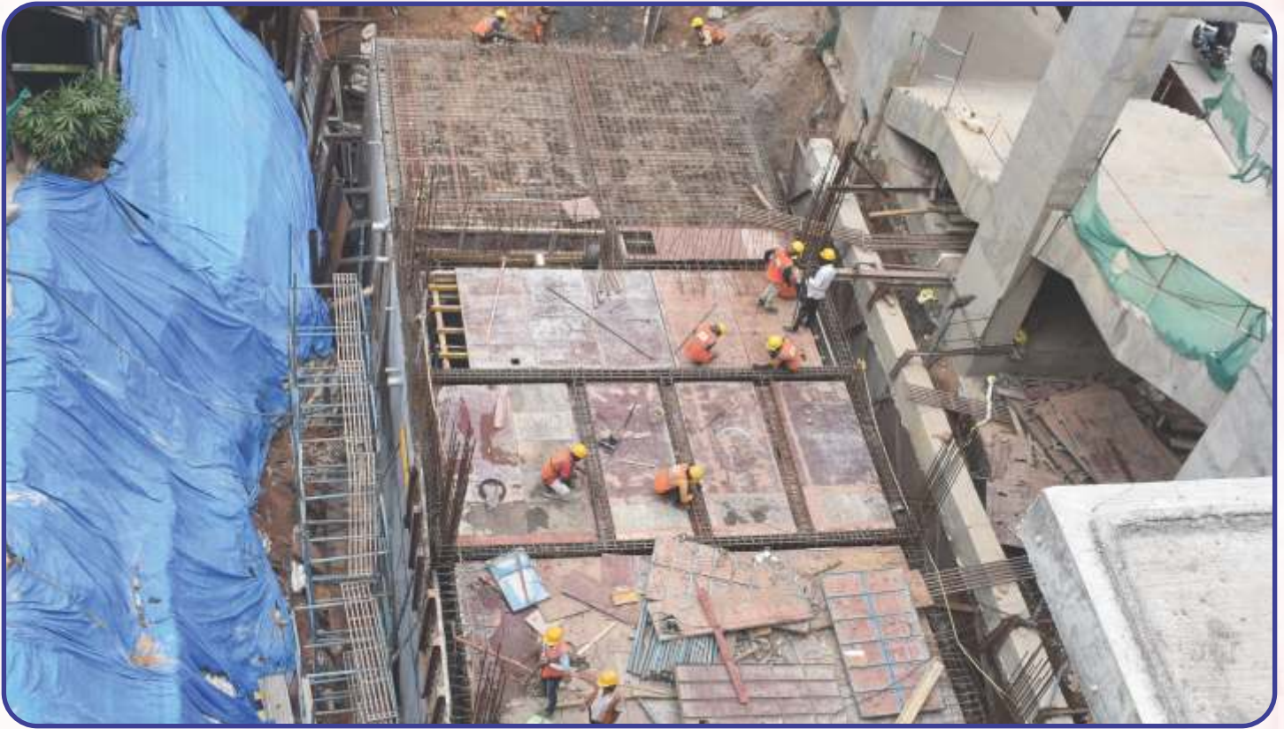
Ongoing works at Jayadeva Metro Station Underground Sump
