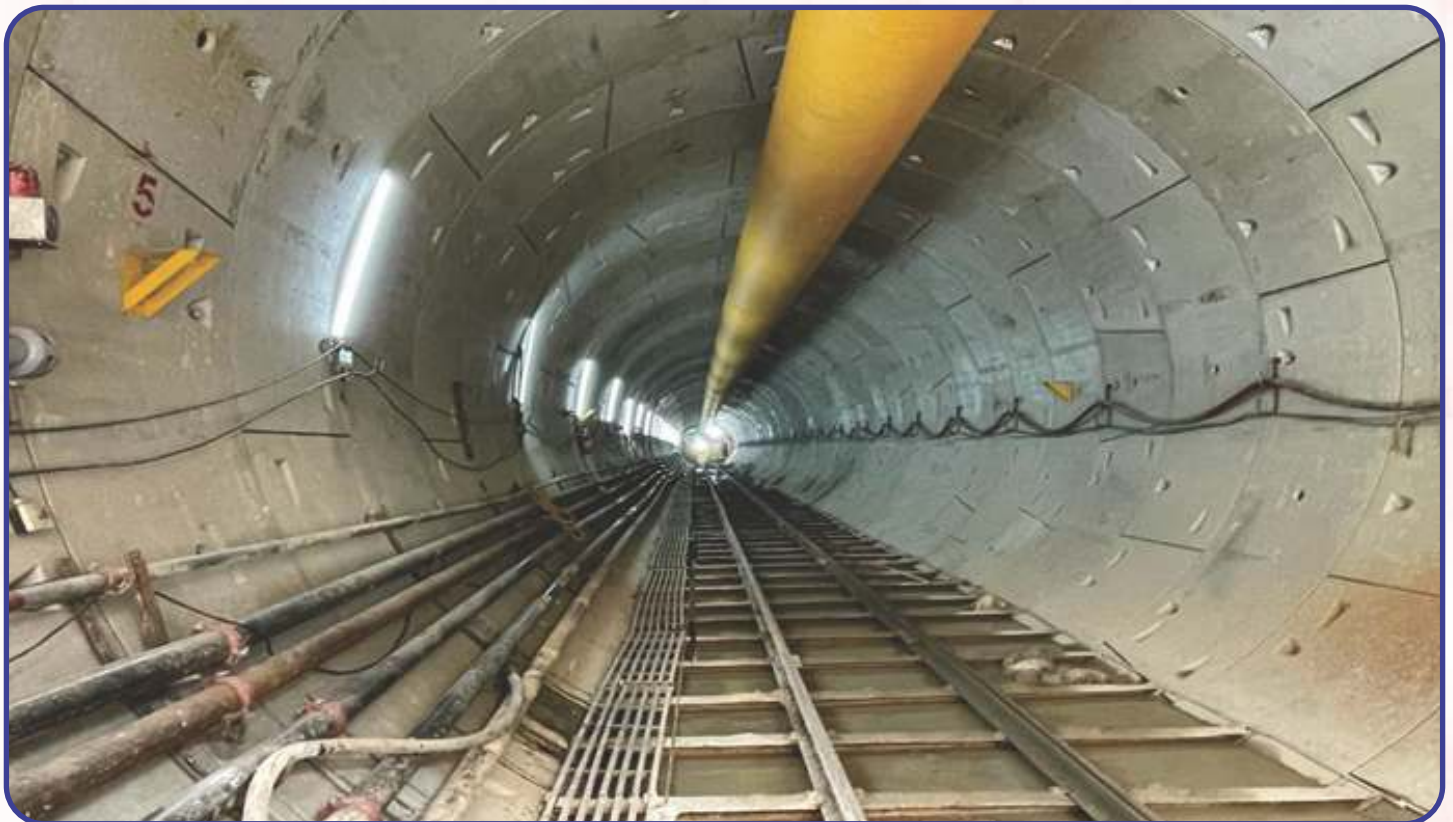
RMS Shaft to Langford Town (South Bound) (TBM Varada)
