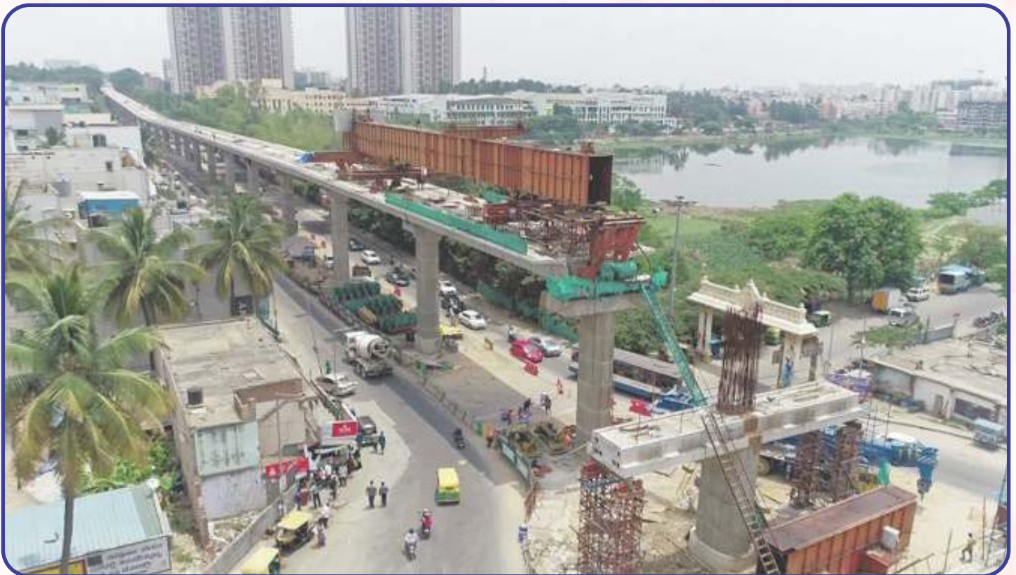
Reach 6 - Elevated : LG2 Dismantling works in progress
