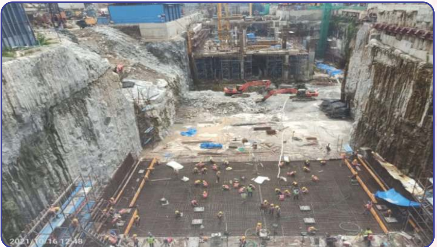
Reach-6 UG View of Cantonment Station works
